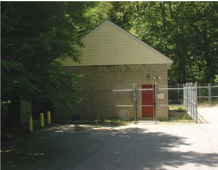
Glen Street Pump Station
