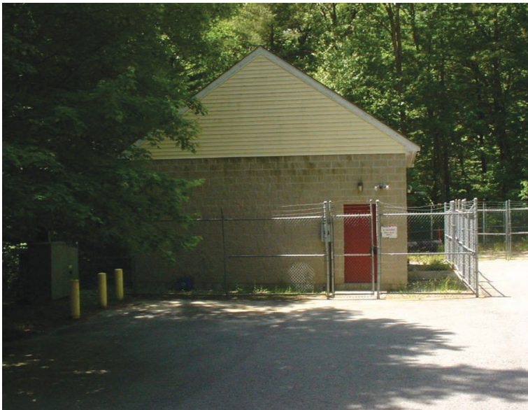
Glen Street Pump Station
