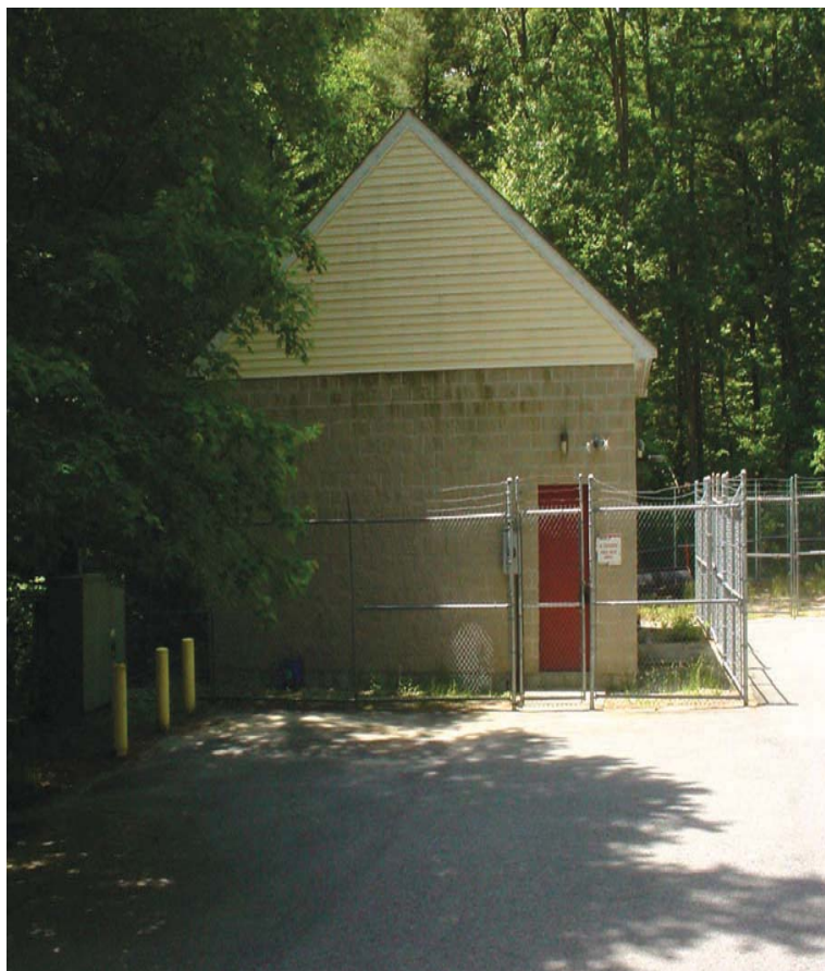
Glen Street Pump Station
