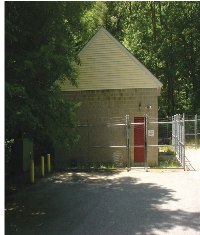
Glen Street Pump Station
